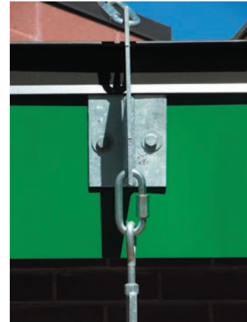
Suspension Cable Connection Plate Detail
